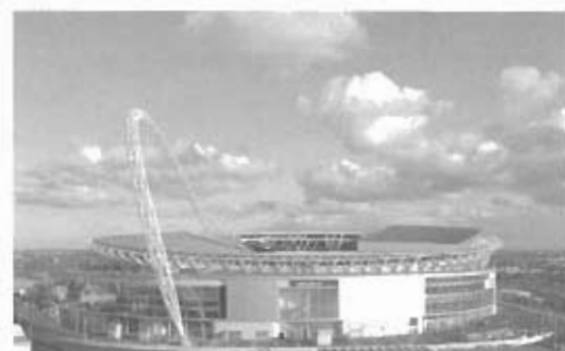
Figure 8. Roof and supporting arch - Case D
